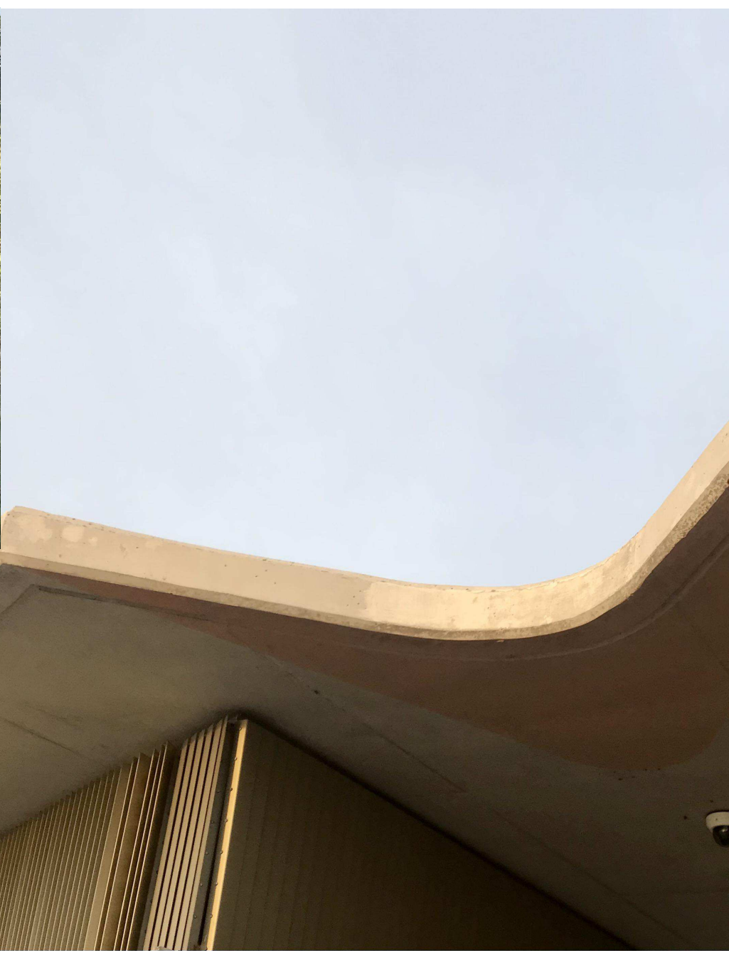
CURVED CONCRETE ROOF
