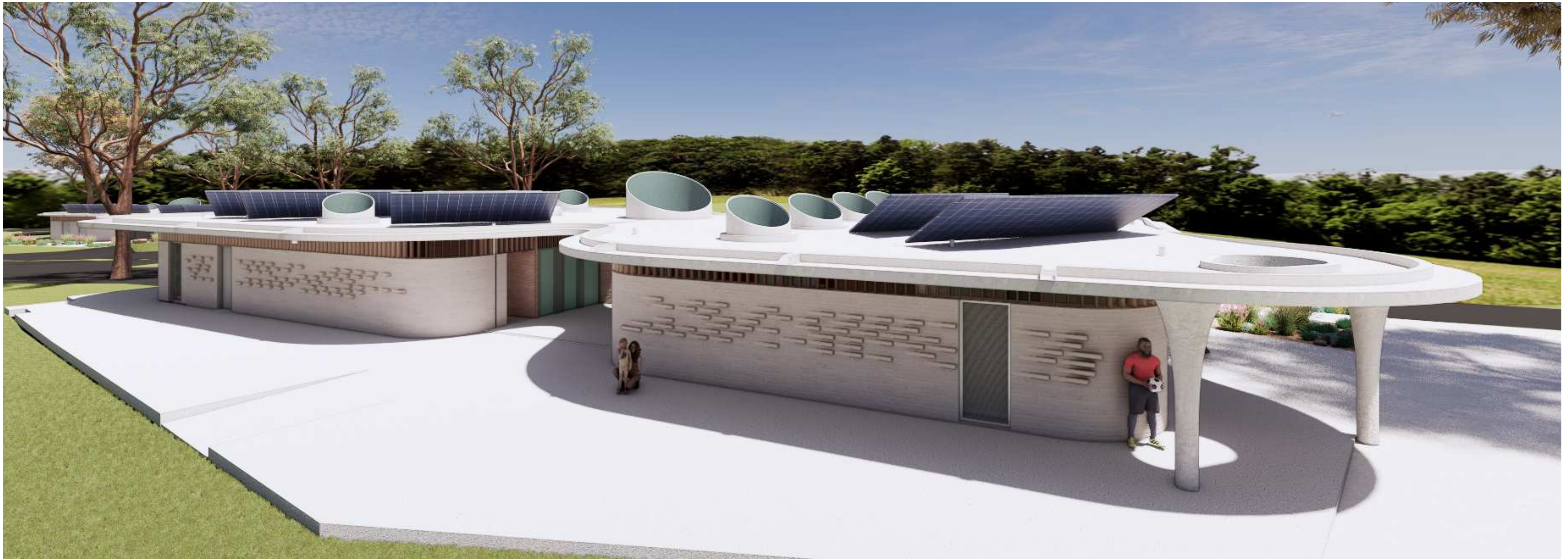
1 BUILDING 2 - AERIAL VIEW WITH BUILDING 3 BEYOND 1:1
