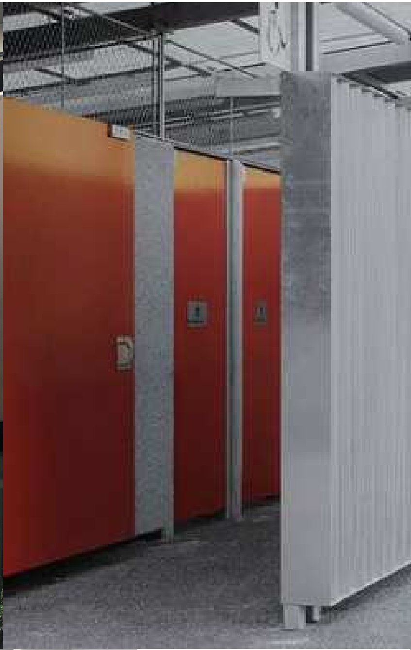
COLOUR FEATURE TO DOORS
