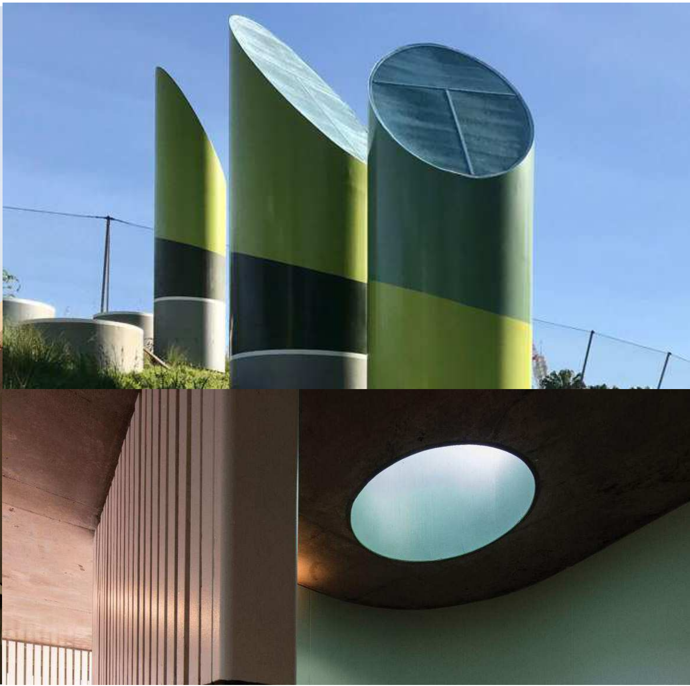
SKYLIGHT CUT-OUTS AND 'TUBES' TO CONCRETE ROOF
